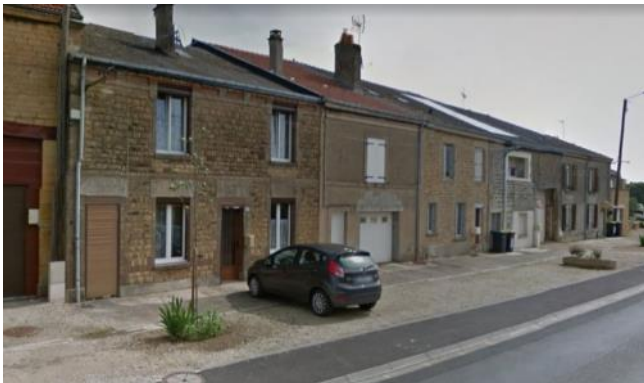
Figure 4.19 Centre ancien rural du village de Vrigne-Meuse (source Google street view)
